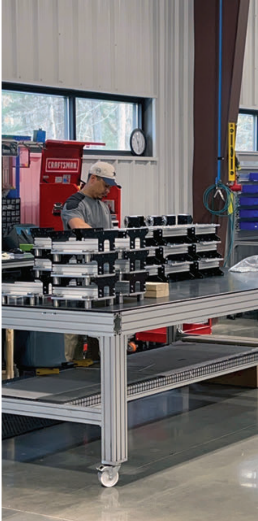
Modular belt conveyors ready for electric car battery line.
