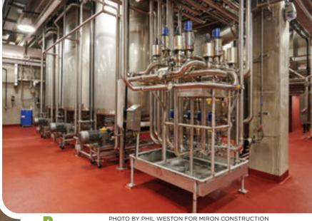
Top: The ground floor level of the Proliant plant contains 3,500-gal crystallizers. Right: At the 28-ft level is Proliant's milling and sifting area, where the top of the vacuum filter receiver and vacuum blower are visible.
