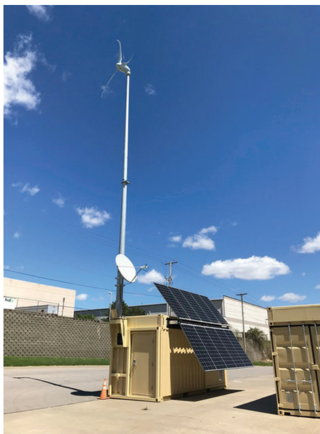
↑ The pod features retractable solar panels and a wind turbine. (Credit: Vaccine Pods)
