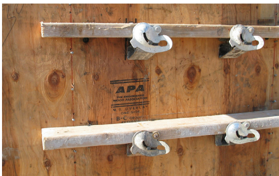
The APA trademark signifies the manufacturer's commitment to a rigorous program of quality verification and testing.
