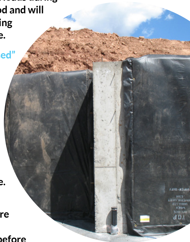
Protect concrete surfaces and corners from cold weather by ensuring all surfaces are covered.
