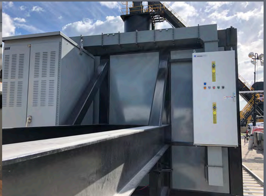
OUTDOOR-RATED KNIFE SWITCH (LEFT) & MAIN DISCONNECT (RIGHT)
