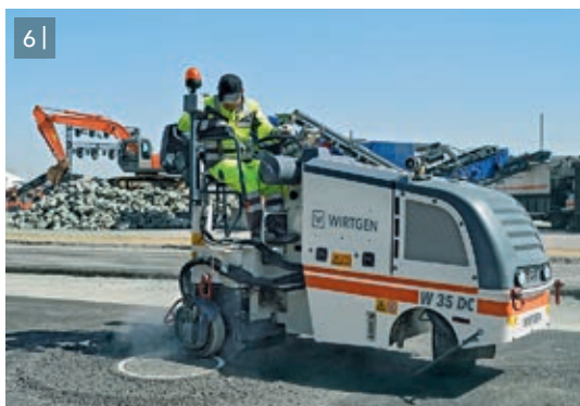
6 | Precise milling around road fixtures without the need for additional manual reworking.
