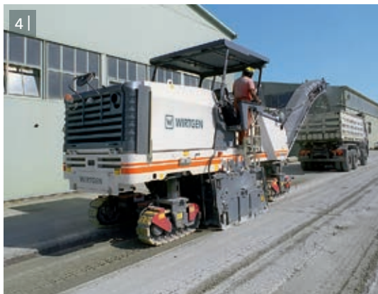
3 | Removing surface deformations by means of fine milling.
