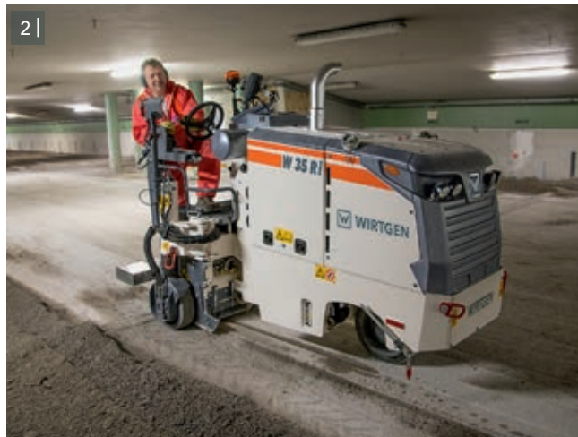
2 | Milling operation in a building with low ceiling height and a floor of limited bearing capacity.
