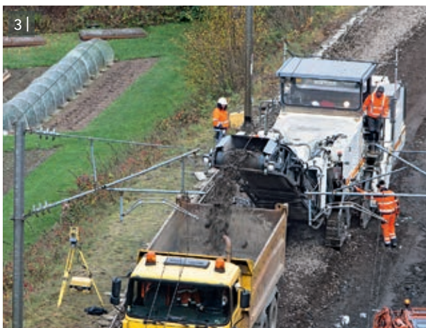
3 | Using laser or 3D control in the milling process complies with the high standards that are applicable in Western Europe.
