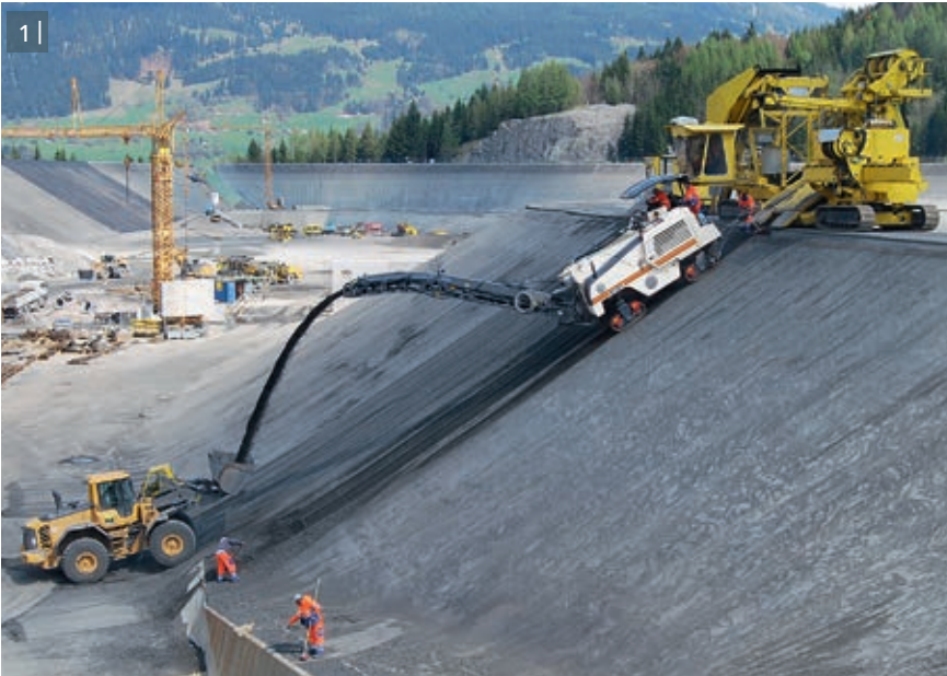
1 | Milling on the steep slope of a water reservoir.
