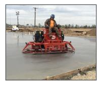
The HP205 riding trowel, features twin 37 hp Kohler EFI gasoline engines. These machines are workhorses built for concrete professionals to deliver maximum horse power with electronic fuel injection. Utilizing torque converter clutches, they provide excellent low speed torque for low speed float panning and superior high rotor speed for finishing concrete.
