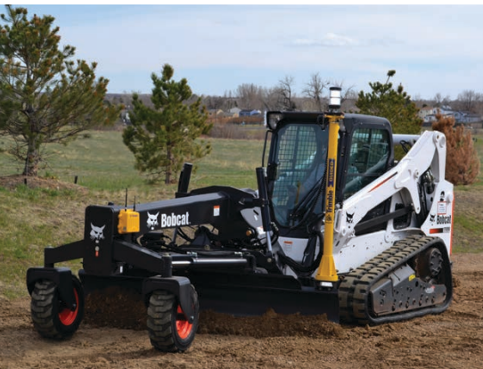
Bobcat with HD Grader Attachment and Trimble GCS900 Grade Control System with Universal Total Station
