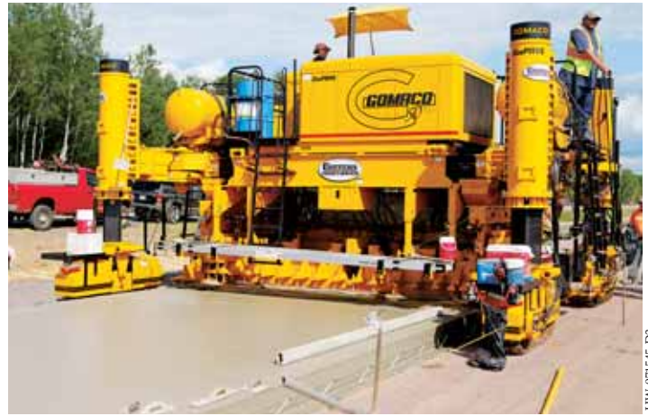
The modular frame on GOMACO's GP3 has telescoping capabilities up to seven feet (2.13 m) on each side.
