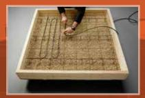
Use the included wire ties to secure the heating cable to a properly installed welded wire mesh or rebar reinforcing system.
