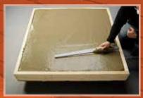
Complete final pour and level concrete to complete the installation.
