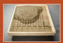
Pour concrete directly over heating cables.
