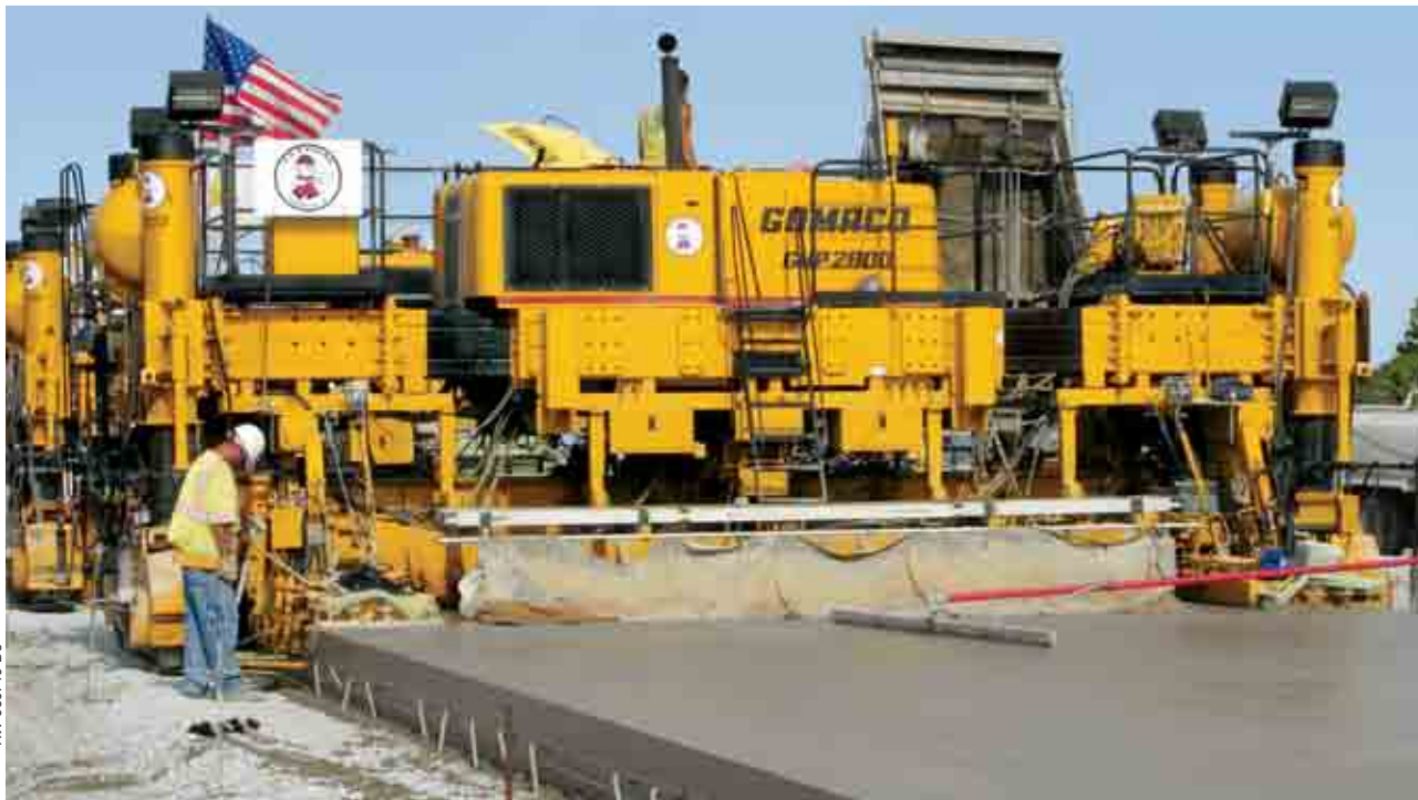
The four-track GHP-2800 is paving 24.6 ft. (7.5 m) wide and 11 in. (279 mm) thick on this mainline paving project in Baja, California.
