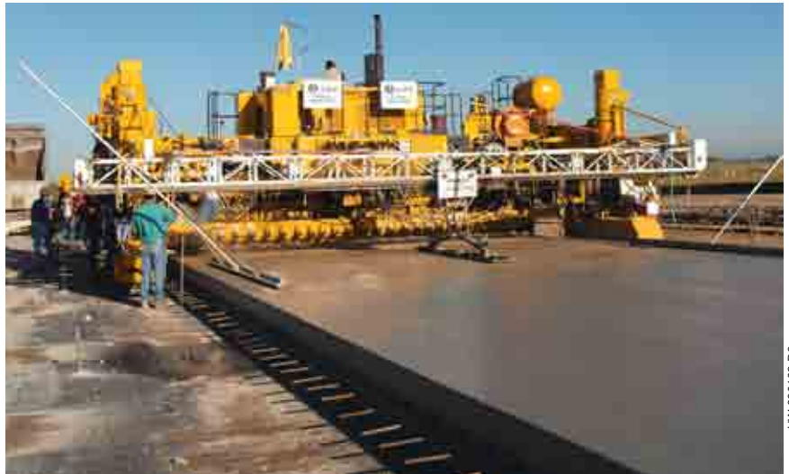
The GHP-2800 easily handles this large airport project in Detroit, Michigan. The runways were slipformed in six 25 ft. (7.62 m) wide lanes, with side bar insertion, for a total runway width of 150 ft. (45.7 m). The depth of the runways were 17 in. (432 mm). Each of the lanes were 10,000 ft. (3048 m) long. The GHP-2800 was equipped with edge slump control, providing the superior GOMACO edge, which is a requirement for airport paving.
