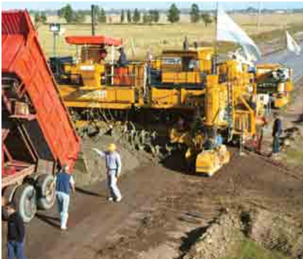
Peak production on this mainline paving project in Argentina was 5912 ft. (1802 m) in an 11-hour shift. The GHP-2800 was equipped with an IDBI dowel bar inserter. High-production paving was achieved while slipforming a 24 ft. (7.32 m) wide by 8.27 in. (210 mm) thick slab.
