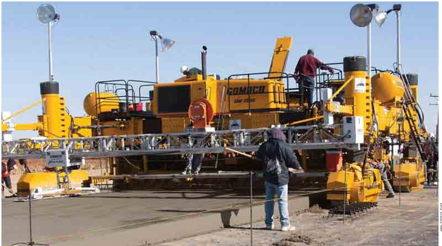
The four-track GHP-2800 is paving 24.6 ft. (7.5 m) wide and 11 in. (279 mm) thick on this mainline paving project in Baja, California.
