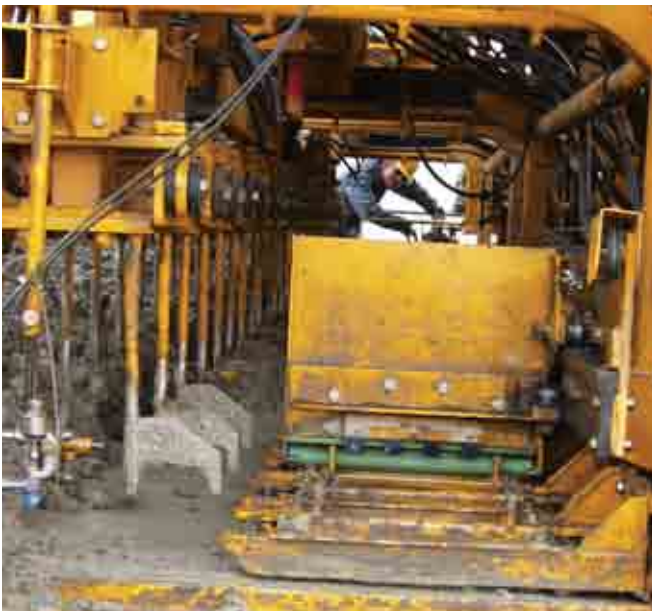
Peak production on this mainline paving project in Argentina was 5912 ft. (1802 m) in an 11-hour shift. The GHP-2800 was equipped with an IDBI dowel bar inserter. High-production paving was achieved while slipforming a 24 ft. (7.32 m) wide by 8.27 in. (210 mm) thick slab.
