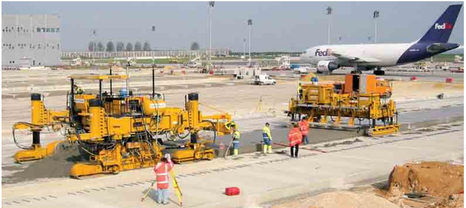
Stringless Paving on Airport near Paris, France
