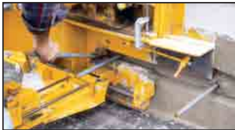
Female keyway with hydraulic side bar insertion and vibration to the bar.
