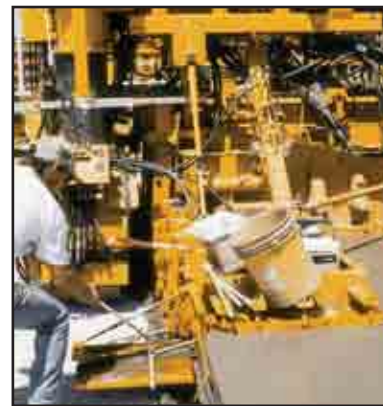
Trailing Form With Manual Bar Insertion
