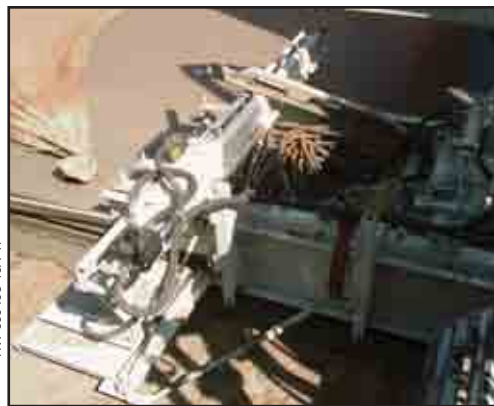
Trailing Form With Air-Powered Bar Insertion
