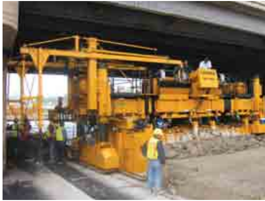
Front view of the GHP-2800 as it paves under the bridge overpass with the hydraulic gantry system retracted.
