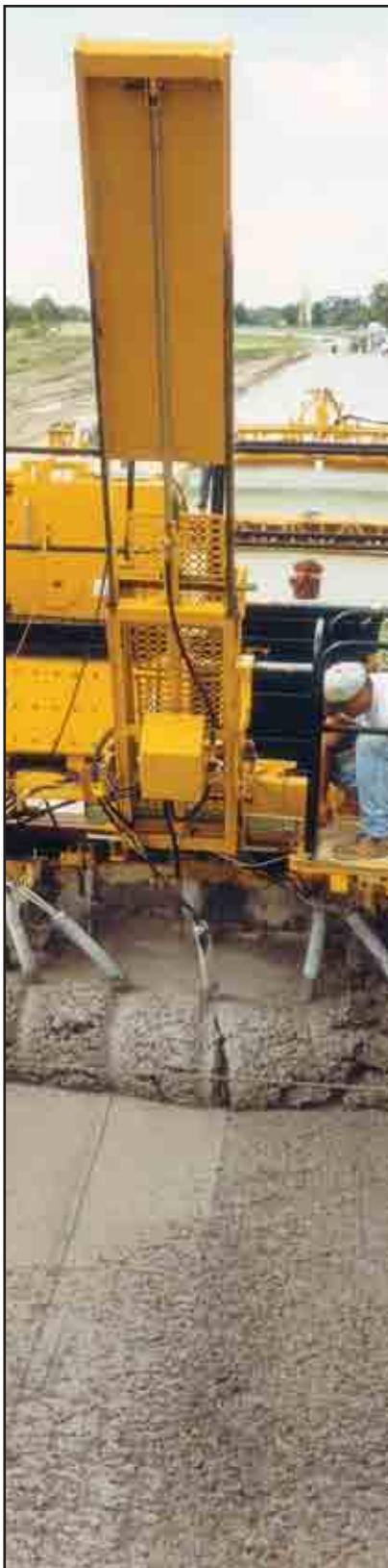
Female keyway with hydraulic side bar insertion and vibration to the bar.
