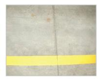
After 21 years of service, we are very pleased with the performance of this floor. Every piece of equipment and material delivered to this building has crossed this joint.
