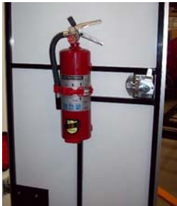
Fire extinguisher inside rear door
