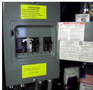
Main Breaker Panel
