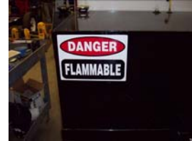
“Danger” front of fuel tank
