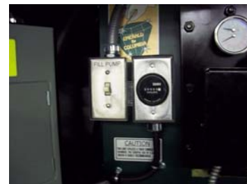
Fill Pump Switch and Hour Meter
