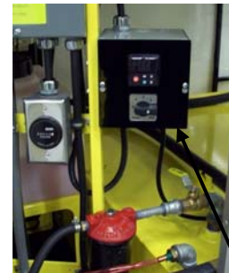
Digital Return Tem- perature Display and rooftop beacon control
