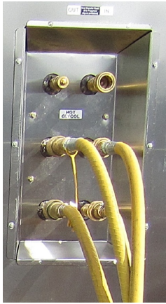
31: Hoses Connected to CHH-980
