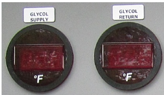
17: Glycol Temperature Gauges
