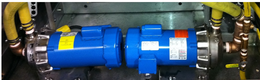
8: Fluid circulation Pumps
