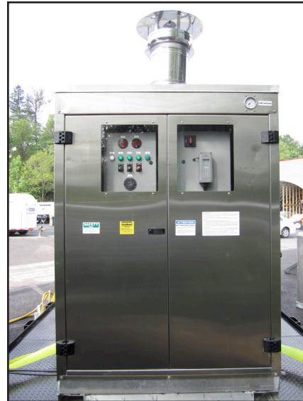
2: CHH-980, Burner End
