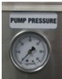
28: Pump Pressure Gauge (PSI)
