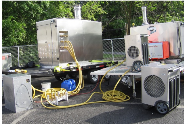
32: Fancoils Connected to CHH-980 Unit
