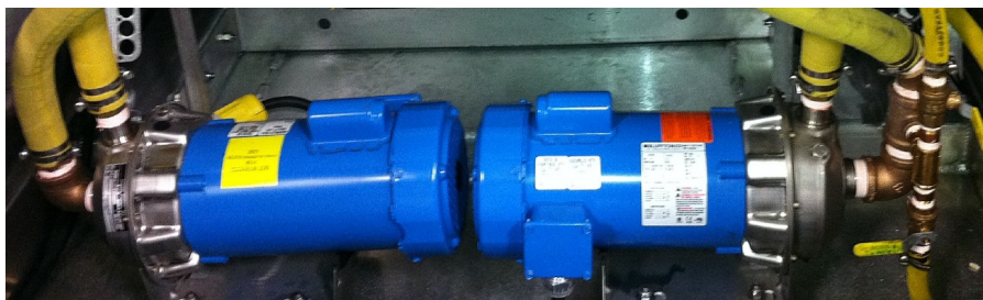
8: Fluid circulation Pumps
