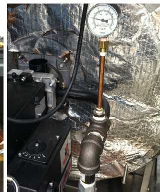
29: Gas Train & Pressure Gauges ("WC)
