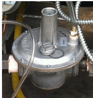
5: Internal Pressure Regulator
