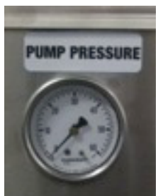
28: Pump Pressure Gauge (PSI)
