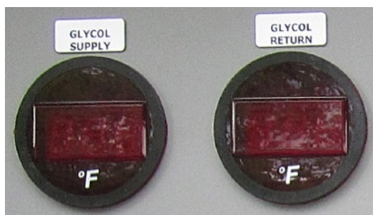
17: Glycol Temperature Gauges
