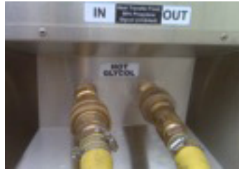
28: Hoses Connected to CHH Unit
