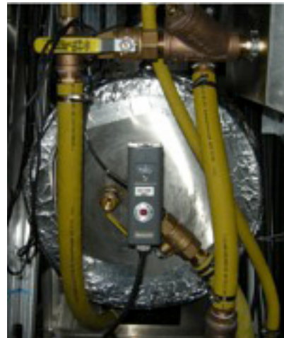
33: HTF Circuit Valves, Y-strainer & High Temp. Limit
