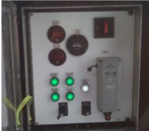
8: Control Panel, Outer
