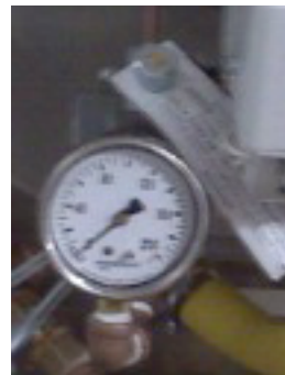
26: Fuel Oil Pressure Gauge (PSI)
