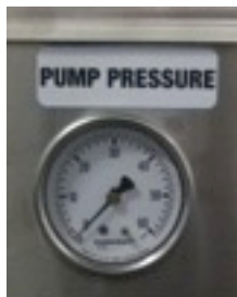
25: Pump Pressure Gauge (PSI)
