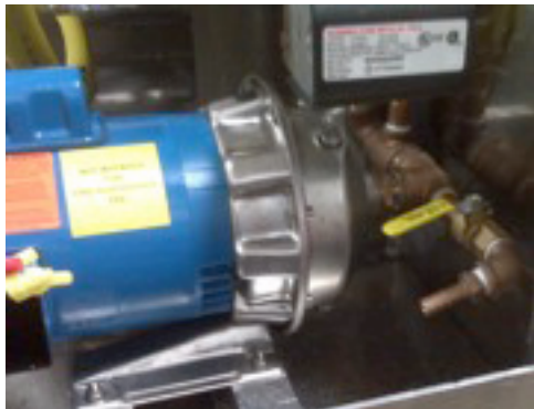
6: Fluid circulation Pump
