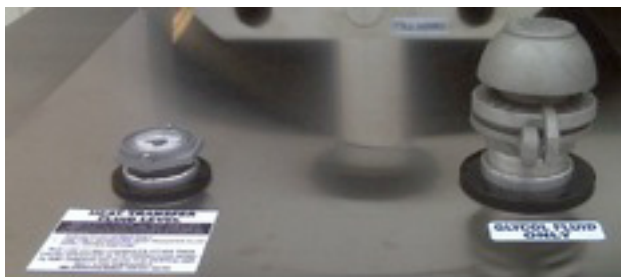
32: HTF Level Gauge & Vented Filler Cap
