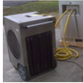
29: Fancoil Connected to CHH Unit
