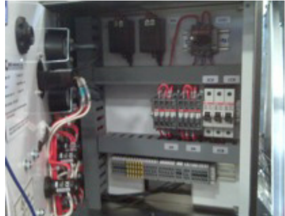
9: Control Panel, Inner
