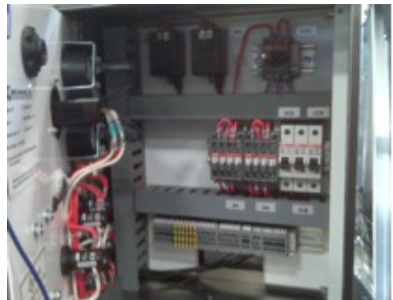
7: Control Panel, Inner
