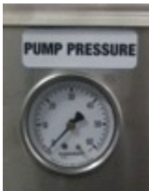
23: Pump Pressure Gauge (PSI)
