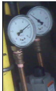
24: Gas Pressure Gauges ("WC)
