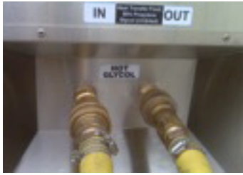
26: Hoses Connected to CHH Unit
