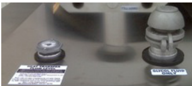
30: HTF Level Gauge & Vented Filler Cap
