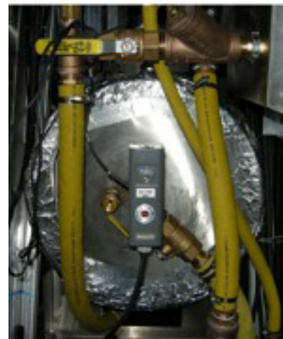
31: HTF Circuit Valves, Y-strainer & High Temp. Limit
