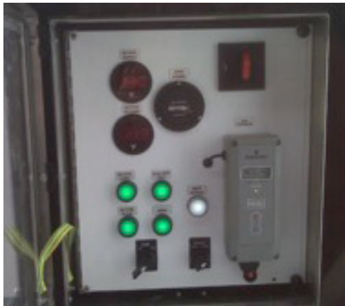
6: Control Panel, Outer
