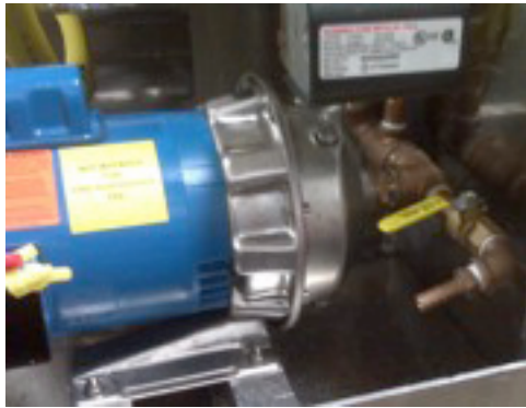
4: Fluid circulation Pump
