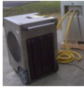
27: Fancoil Connected to CHH Unit
