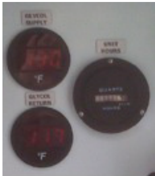
12: Temperature Gauges & Hour Meter
