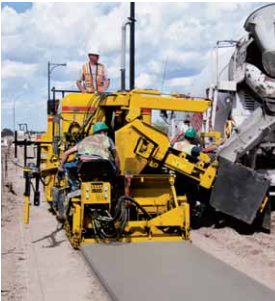
The GT-3200 specifically designed for sidewalks in rehabilitation projects.
