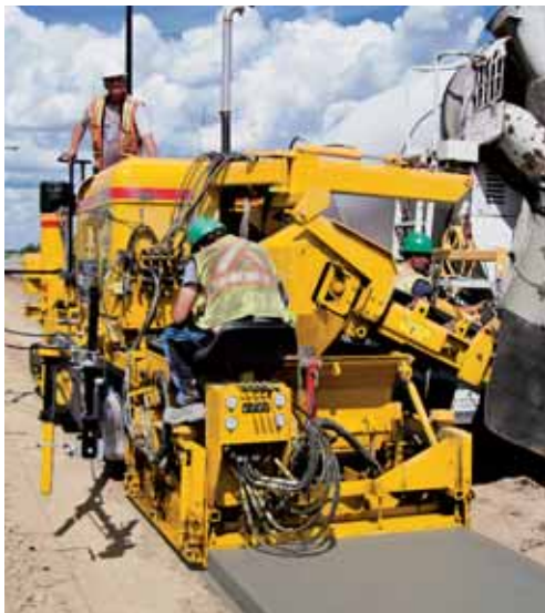
The GT-3200 with a rear-mounted mold for five foot (1.5 m) sidewalk is paving with zero clearance on both sides of the machine.
