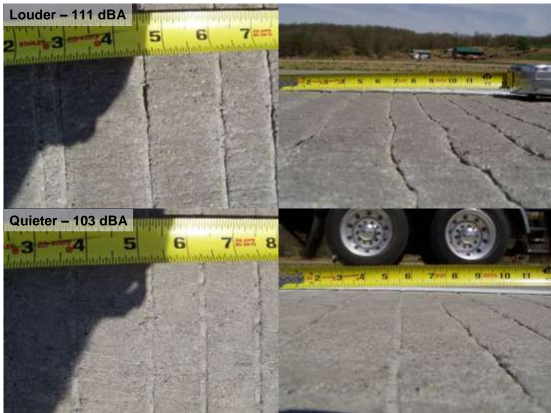
Figure 8. Variability of transverse tined surface and its effect on OBSI noise level.
