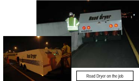
Road Dryer on the job
